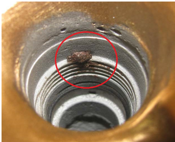
Figure 3. Inspect Nozzle Recess Threads
